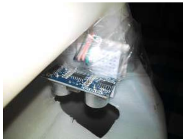
Figure B.2: View of the sensor and connections.
